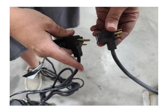
Connect power cords as shown and place sump pump in pit
